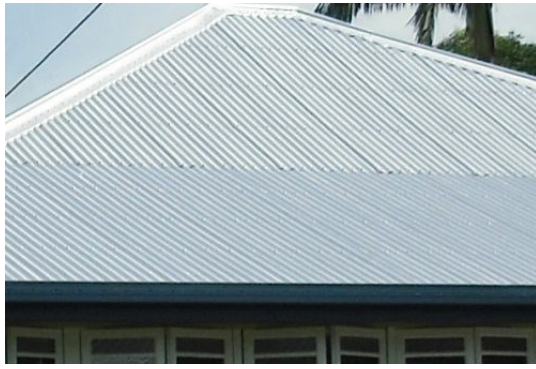
Figure SC6.2.3.22 Corrugated galvanized iron is typical for roofing in Townsville Character buildings
